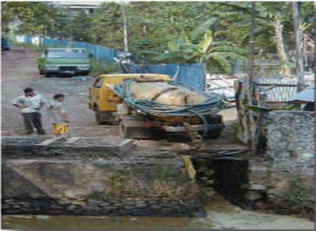
Sewerage System from household directly to public drainase or river without treatment
