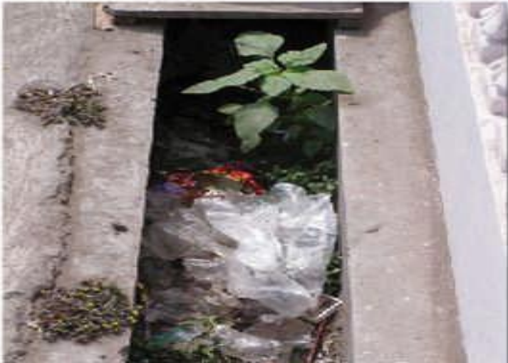
Waste in drainase
